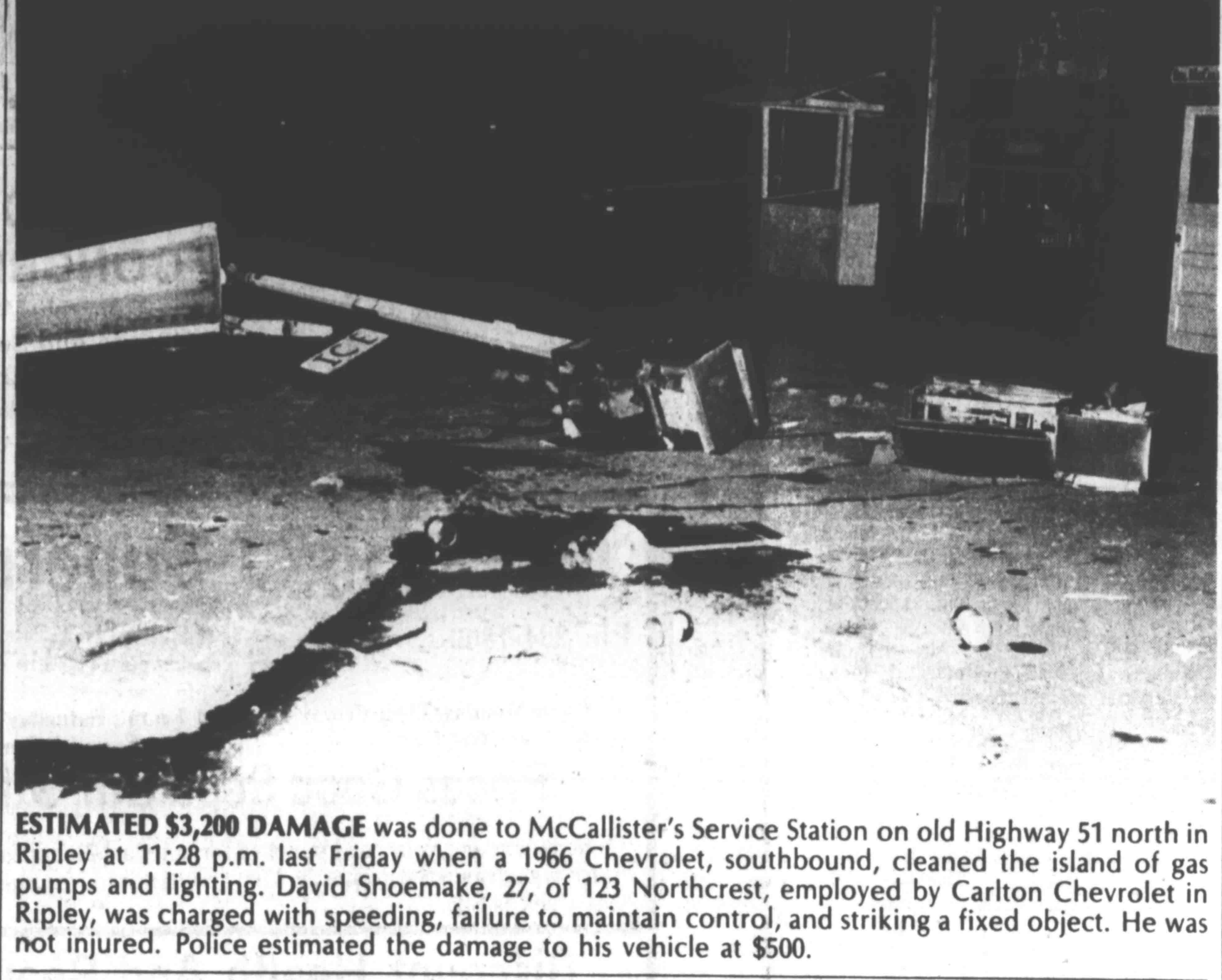
ESTIMATED $3,200 DAMAGE was done to McCallister's Service Station on old Highway 51 north in Ripley at 11:28 p.m. last Friday when a 1966 Chevrolet, southbound, cleaned the island of gas pumps and lighting. David Shoemaker, 27, of 123 Northcrest, employed by Carlton Chevrolet in Ripley, was charged with speeding, failure to maintain control, and striking a fixed object. He was not injured. Police estimated the damage to his vehicle at $500.
