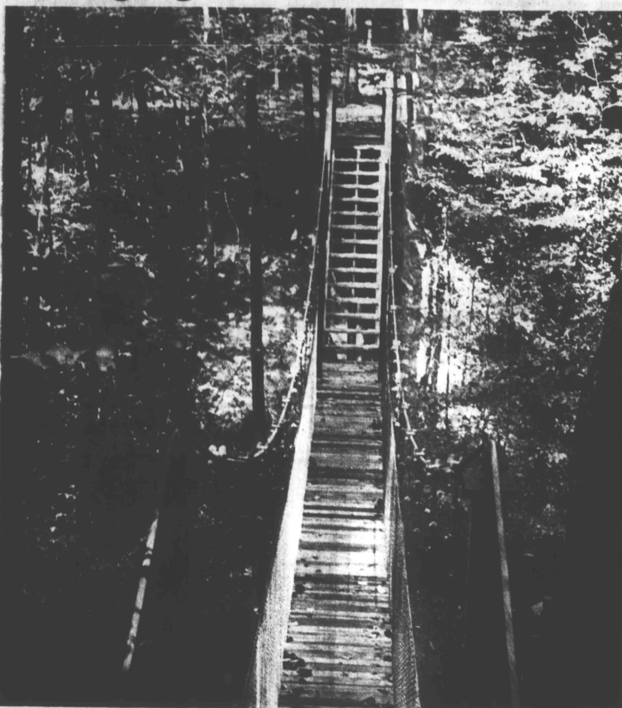
A SUSPENSION BRIDGE HAS BEEN COMPLETED over ravine in Fort Pillow State Historical Area.
